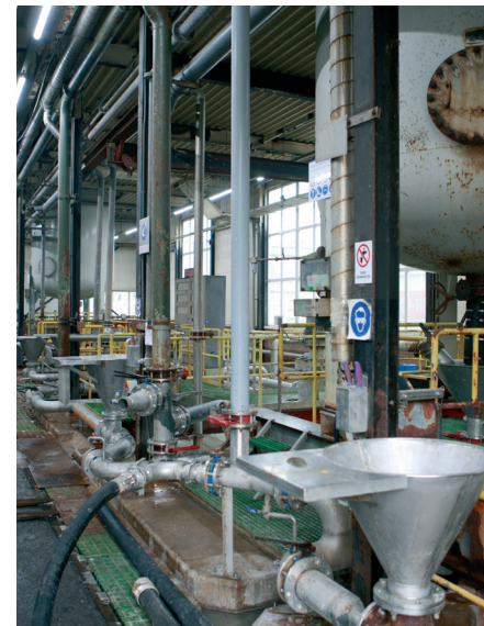
Mud Plant REYM
