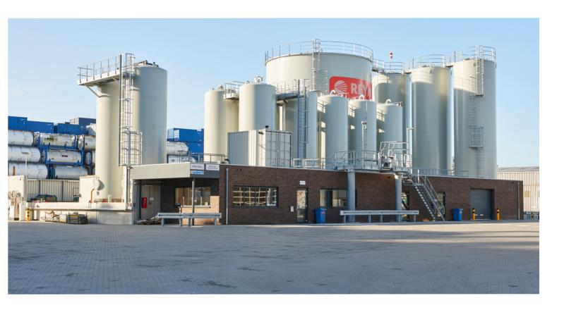
With the help of our WTPs in Rotterdam, Beverwijk, Sittard and Veendam, we are able to offer our customers support at the highest level. At the WTPs, oil, water and solids are separated from each other. The purified water is discharged via the sewage system in the region. Other waste materials are sent to specialistic companies for further processing.
